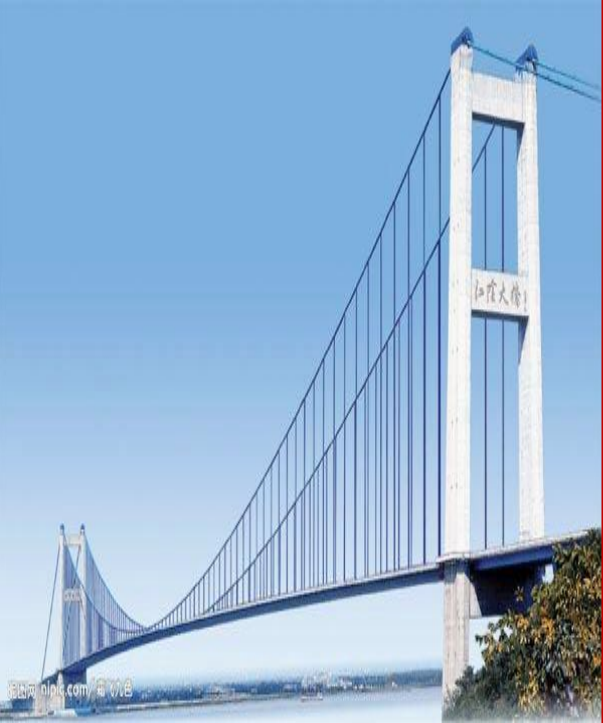
6.Jiangyin Suspension Bridge, China – 1,385 m
