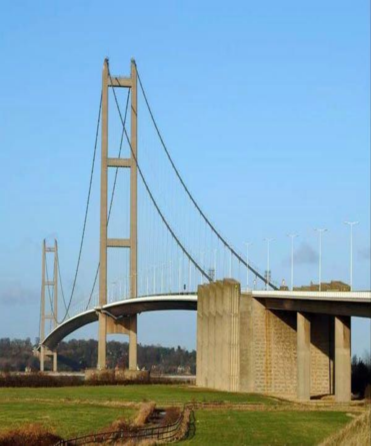
5. Humber Bridge, England – 1,410 m
